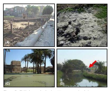
Figure (2): Field photographs showing: (A) water pumping during sewers net instillation, (B): fine particles removed from the aquifer, (C) raw sewage overflows into streets (green color refers to algae cover), and (D) discharge of raw sewage into Qus irrigation canal.
